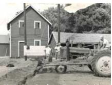
Digging trenches for underground wiring was the first step in an eight-day electrical overhaul of the Hoffman Farm.
