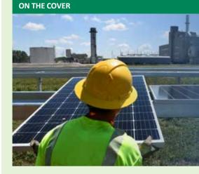
A new single-axis tracking panel is installed at Corn Belt Power Cooperative's new 150-kilowatt solar project at Wisdom Station, Spencer, Iowa. This 600-panel project replaces the space once occupied by the plant's coal pile. Photo taken by Marena Fritzler, marketing director, Corn Belt Power Cooperative. *≸*
